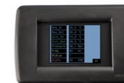
Chiller status display
